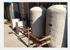
(x 2units = 368 Gallons). With the heaters and storage tanks, the YMCA will get a 582 GPH recovery at the  $80^{\circ}$ F temperature rise typical to Santa Rosa.
